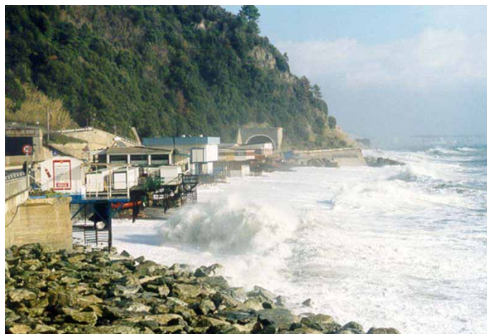
FIGURE 3 View of the beach of Vesima looking eastwards (in February 2000) before the nourishment.
